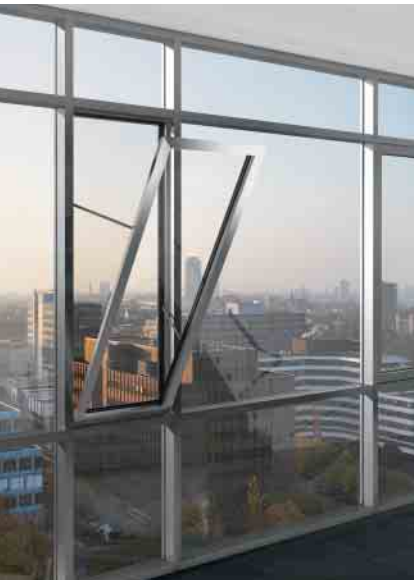
Zugbrücke in Treppenhaus Drawbridge in a stairwell
